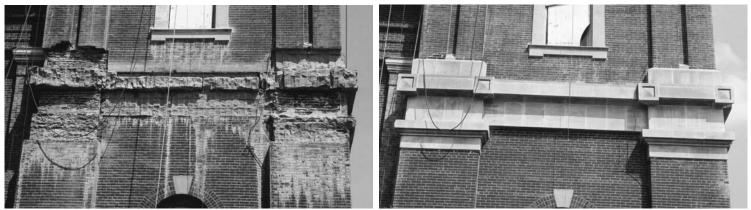
BEFORE: West tower, lower band, facing 11th St. with old, deteriorated sandstone cut back ready for application of new limestone.
