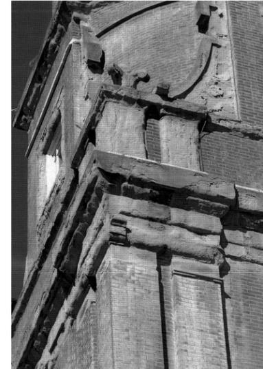
Typical deterioration of stone on corners and horizontal surfaces.
