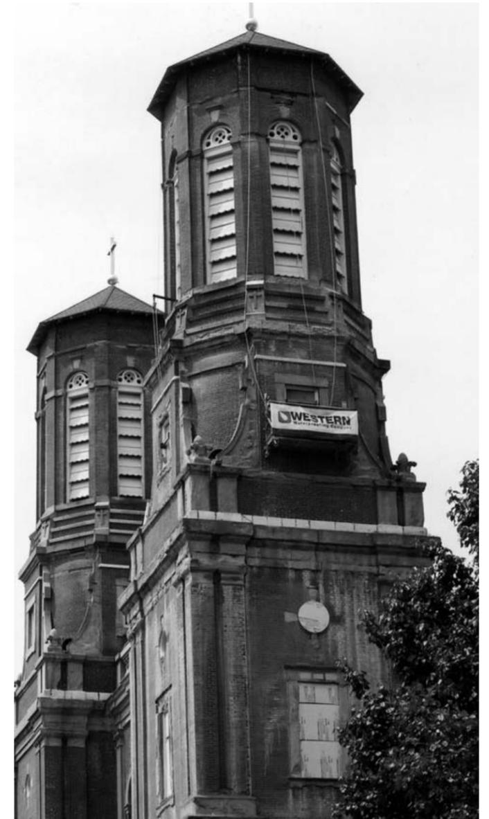
Workers on platform called staging suspended down from top of east tower with cables are in the process of cutting back and removing deteriorated sandstone.
