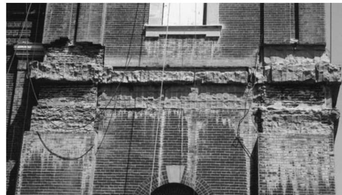
BEFORE: West tower, lower band, facing 11th St. with old, deteriorated sandstone cut back ready for application of new limestone.
